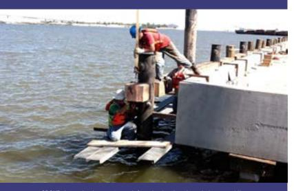
GROUP determined a way to work from land rather than via barges while building this 984-foot-long by 30-foot-wide concrete dock, which gave crews better access to the site and saved the client \$260,000 in operating costs.
