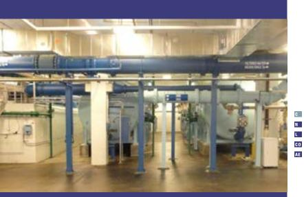
Municipal Builders repurposed 24,780-square-feet of the bottom level of a parking garage into the Edina Water Treatment Plant No. 6, which aids the removal of vinyl chloride from the city's water supply.
