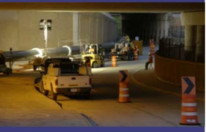
ACI Mechanical successfully re-routed chilled waterlines at George Bush Intercontinental Airport after a 10,000 gallon-per-day leak was discovered in its underground distribution system.
