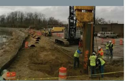
On its first prime contract with the USACE, Kwest Group safely dealt with overhead utilities and underground conflicts while constructing 2,600 traversing feet of customized reinforced concrete floodwalls partially located within 25 feet of surrounding businesses.
