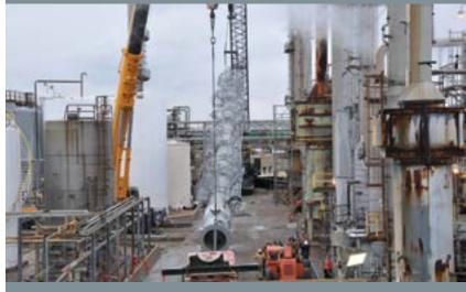
In just eight months, Turner Industries Group completed the design, fabrication, delivery and installation of a 100-ton, 206-foot-long distillation column, including a long, incident-free haul from Decatur, Ala., to Houston.
