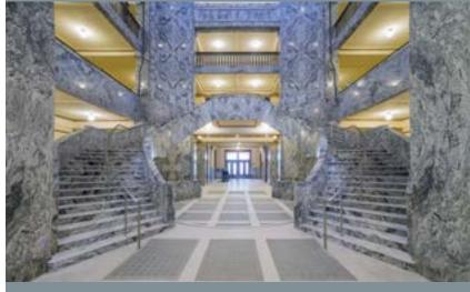
Camarata stepped in to restore historical elements of a 103-year-old courthouse, including refinishing 21,000 square feet of original stone, installing 4,642 square feet of new stone and incorporating 17,545 square feet of matching marble.
