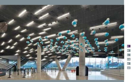
BakerTriangle relied on ingenuity, BIM and robotic total stations to safely create and install an undulating wire mesh ceiling, metal ribbon wall feature and curved escalator "tube" for a LEED Gold science museum.
