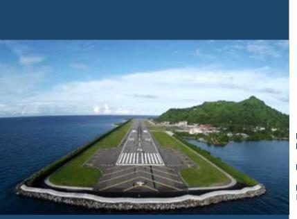
Black Construction Corporation achieved 300,000 manhours without a lost-time incident while rehabilitating a runway at Chuuk International Airport in Micronesia. Fifty thousand tons of aggregates were imported via a break bulk vessel and multiple barge trips were necessary to mobilize heavy equipment and asphalt/concrete.
