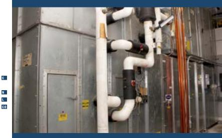
A year of planning and collaboration with all project participants allowed The Cincinnati Air Conditioning Co. to replace three 100-ton central station air handlers in just five 24-hour days, as well as rig large equipment through small openings in this historical transit terminal turned office building.
