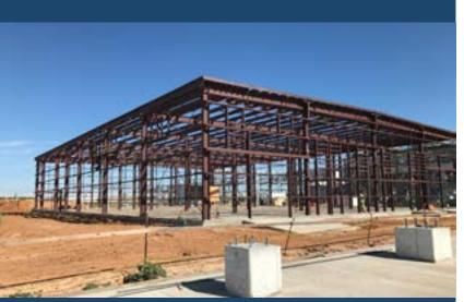
GROUP contractors completed the grassroots construction of a 15,000-square-root, pre-engineered metal motor control center building ahead of its liquidated damages deadline despite materials delays, site constraints and extraordinary concrete finishing requirements. Through it all, the deadline for the building remained fixed.
