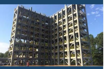
Brasfield & Gorrie's role on this unique project involved constructing two NASA launch system stands designed to test the largest ever liquid oxygen/liquid nitrogen fuel tanks that will help send astronauts on deep space missions and eventually to Mars.
