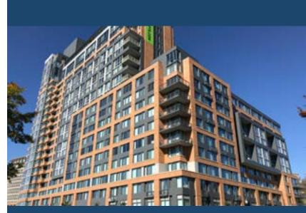
Brickwork starts and stops at various heights throughout this 25-story luxury apartment building—causing difficult access across four scaffold systems for Telligent Masonry, which completed the bulk of the work in five months.
