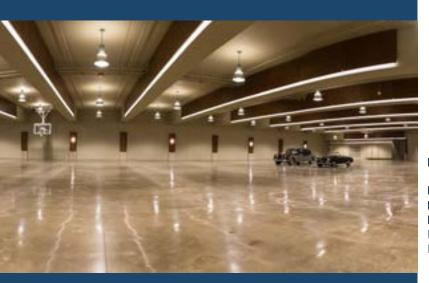
Adolfson & Peterson Construction built a 73-vehicle underground parking garage concrete beams-with a span of 105 feet at the widest point-that are clad with oak veneer panels and backlit with LED strip lighting.
