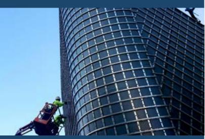
KENPAI's work on this science museum elevated industry standards through the extensive use of 3-D parametric modeling, the iterative translation of the precise location of x-q-z coordinates for each construction layer, and the installation and grouting of more than 400,000 circular tiles.
