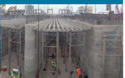
Cajun worked nearly 112,000 incident- and injury-free manhours while installing 9,625 cubic yards of structural concrete—including a multi-leveled cooling towe that required a specially engineered sheet pile shoring system—to meet CF Industries' capacity expansion schedule.
