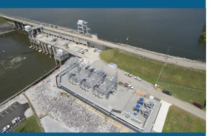
$\ensuremath{\mathsf{M}}$  & D Mechanical Contractors installed two high-capacity blowers and the stainless steel piping necessary to transport air below the Neely Henry Dam, effectively raising the dissolved oxygen content in the water to support aquatic life.
