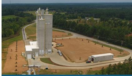
Cobb Vantress Inc. contracted The Weitz Company to design-build a state-ofthe-art poultry feed processing facility in Joanna, South Carolina, that has a manufacturing capacity of 2,000 tons per week for grain storage, grinding, mixing, pelleting and cooling.
