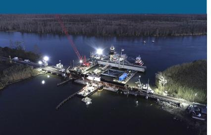
Extreme coordination and planning were required for Brasfield & Gorrie to meet the accelerated schedule to replace a railroad swing span with a new 550,000-pound span, all performed over water and with a rail shutdown of only 14 hours.
