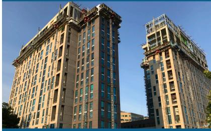
Telligent Masonry safely installed approximately one million oversize bricks on The Signature ahead of schedule, requiring several different crews and multiple scaffold systems. Substantial completion of the skin on the 23-story luxury apartment building's two towers was done in just six months.
