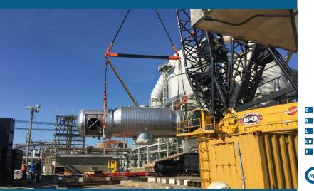
To increase operating capacity and overall efficiency at the Olin Blue Cube Operations facility, Cajun was charged with the demolition, removal and replacement of a 500,000-pound heat exchanger located within a highly congested unit.
