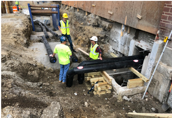
Figure 2. Installing Boiler, Pipe Out of Tunnel
