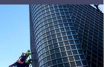
KENPAT's work on this science museum elevated industry standards through the extensive use of 3-D parametric modeling, the iterative translation of the precise ocation of x-q-z coordinates for each construction layer, and the installation and prouting of more than 400,000 circular tiles.
