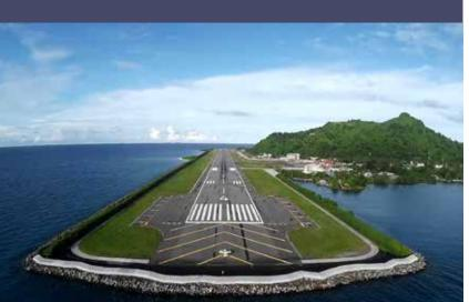
Black Construction Corporation achieved 300,000 manhours without a lost-time incident while rehabilitating a runway at Chuuk International Airport in Micronesia. Fifty thousand tons of aggregates were imported via a break bulk vessel and multiple barge trips were necessary to mobilize heavy equipment and asphalt/concrete.
