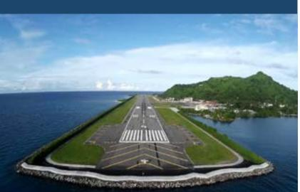
Black Construction Corporation achieved 300,000 manhours without a lost-time incident while rehabilitating a runway at Chuuk International Airport in Micronesia. Fifty thousand tons of aggregates were imported via a break bulk vessel and multiple barge trips were processary to mobilize beauty equipment and asphalt/concrete.
