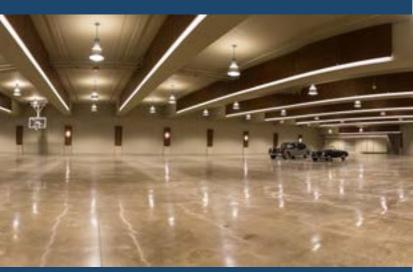
Adolfson & Peterson Construction built a 73-vehicle underground parking garage with a full-length basketball court. The roof consists of cast-in-place post-tension concrete beams—with a span of 105 feet at the widest point—that are clad with oak veneer panels and backlit with LED strip lighting.
