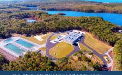
Methuen Construction used dissolved air flotation clarification, horizontal directional drilling and critical path method scheduling to finish this water treatment plant on time while meeting stringent state and federal environmental regulations.
