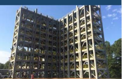
Brasfield & Gorrie's role on this unique project involved constructing two NASA launch system stands designed to test the largest ever liquid oxygen/liquid nitrogen fuel tanks that will help send astronauts on deep space missions and eventually to Mars.
