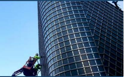
KENPAT's work on this science museum elevated industry standards through the extensive use of 3-D parametric modeling, the iterative translation of the precise location of x-q-z coordinates for each construction layer, and the installation and grouting of more than 400,000 circular tiles.
