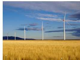
The Judith Gap Wind Energy Center in Montana is comprised of 90 GE 1.5-MW turbines, for a total capacity of 135 MW
